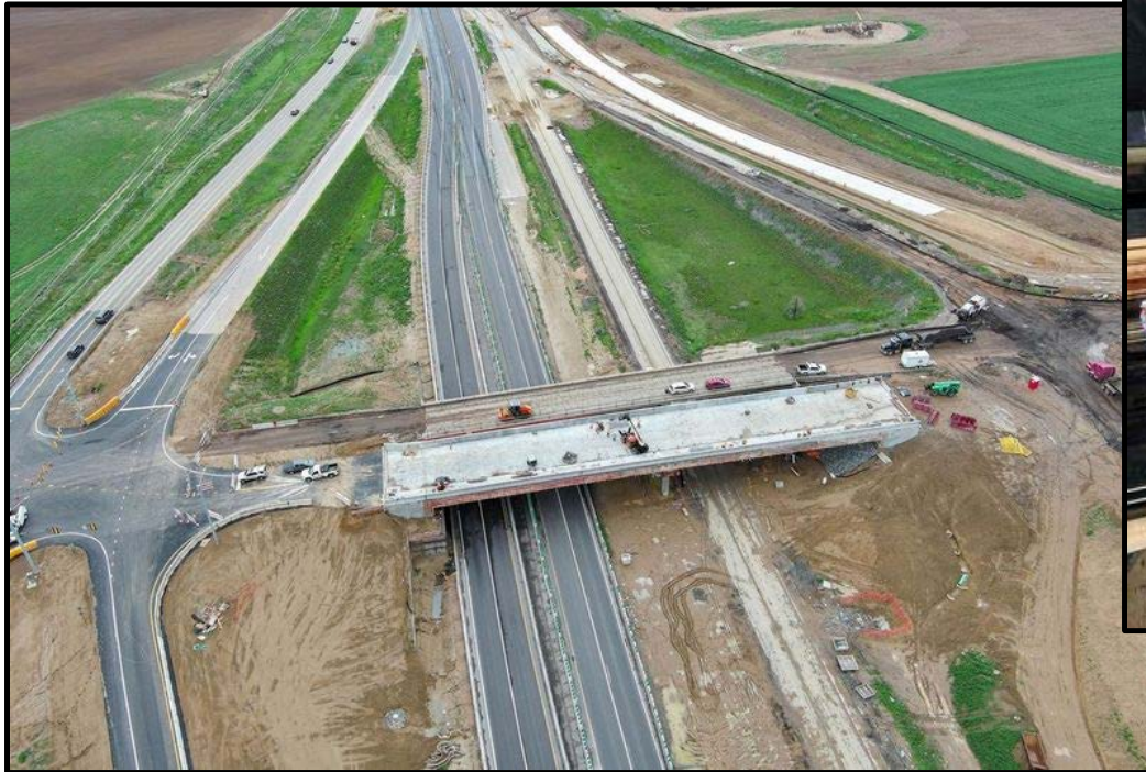
New Bridge Construction - Winter 2024/2025
