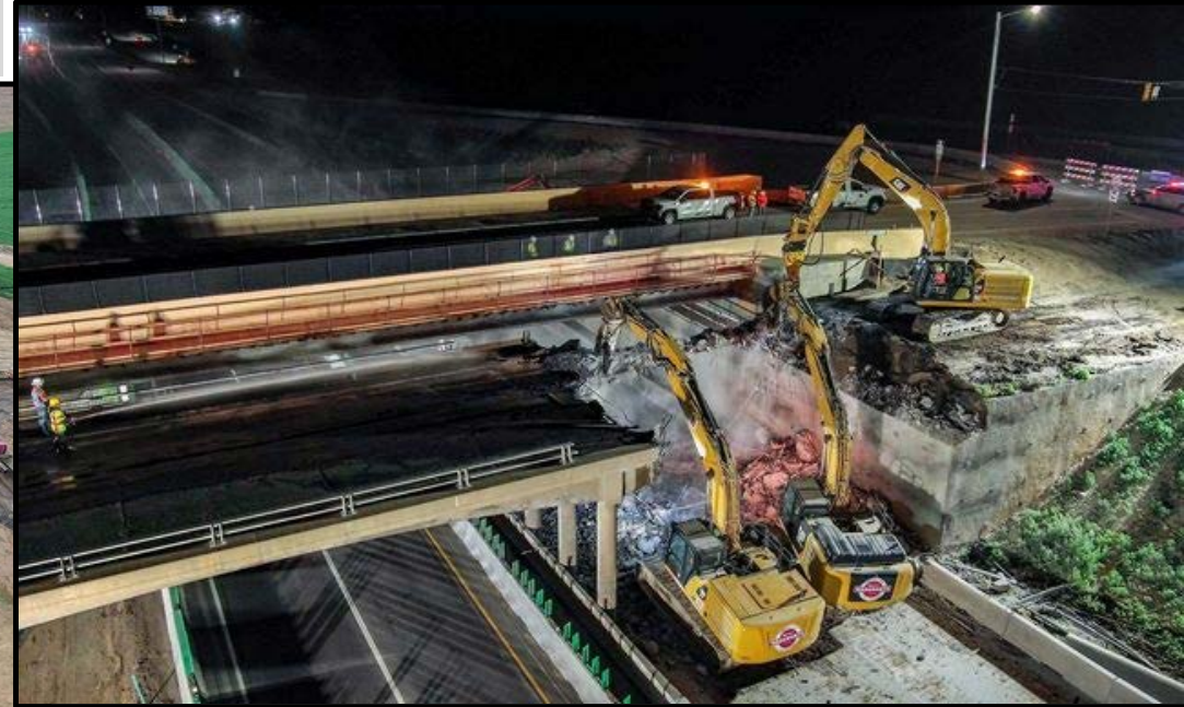
Old Bridge Demolition – June 2025
