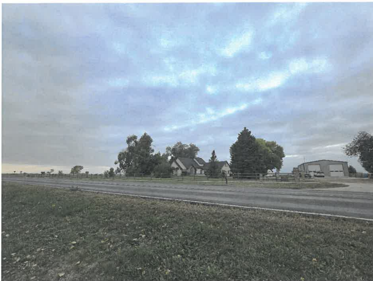
Exhibit C – CR-7 Looking South: View toward proposed entrance; limited safe queue space and exit from CR-7, limited nighttime safety.
