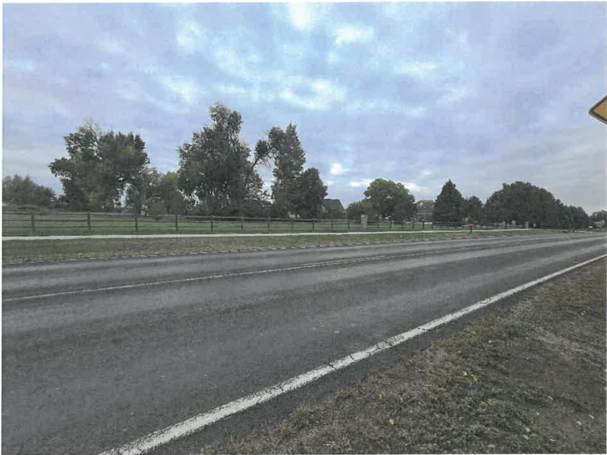
Exhibit B – CR-7 Looking North: Two-lane road, no shoulders/turn lanes. There is no room or easement to widen CR-7 to allow for safer travel.
