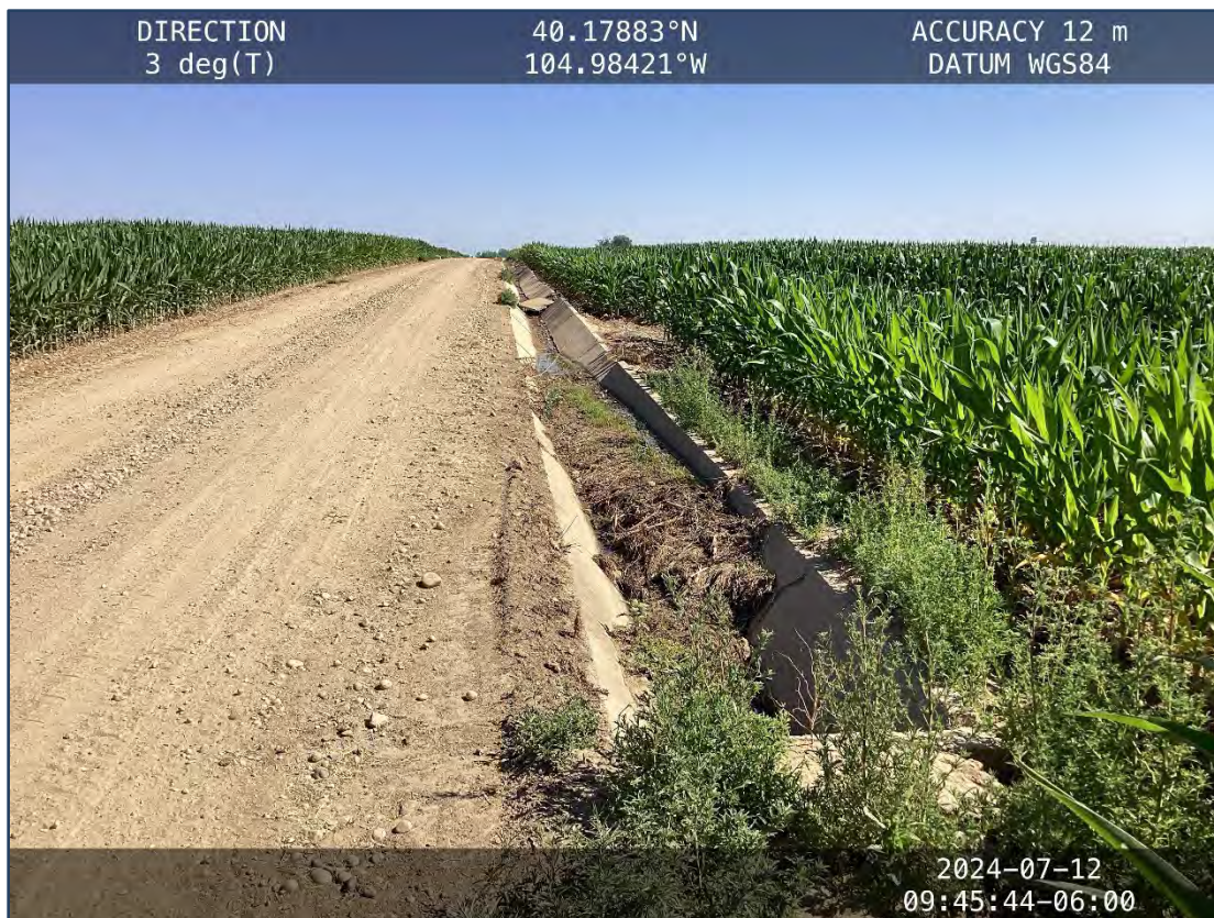
Photograph 7. Looking north along concrete-lined irrigation ditch. Despite presence of sediment/soil, the ditch does support an OHWM.
