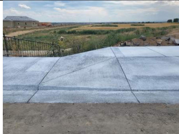
Concrete (Joint alignment)
