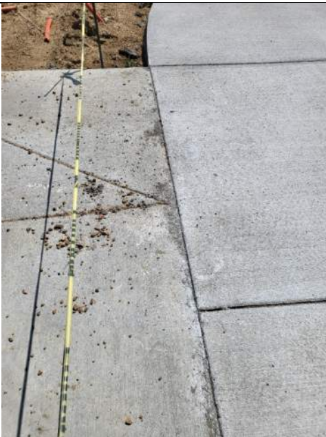
Concrete Clean Up
