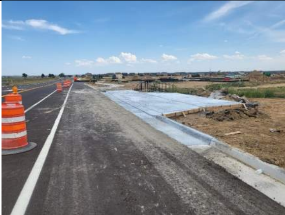
Concrete (Joint alignment)
