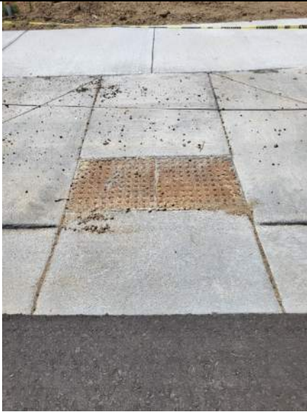
Concrete Clean up/seal all ADA ramps
