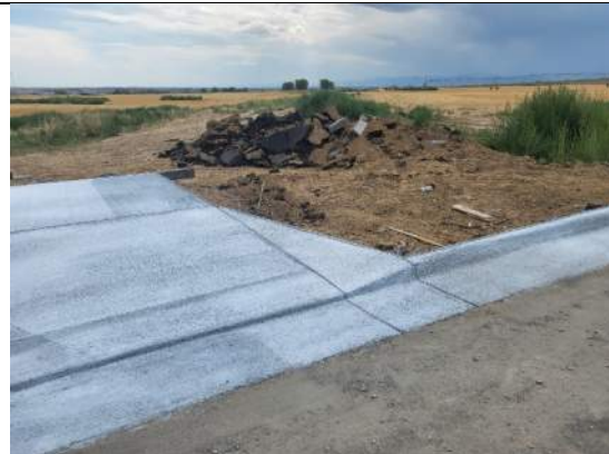
Concrete (Joint alignment) Backfill/Cleanup
