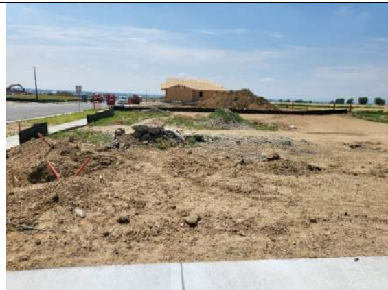
Utilities Exposed/Clean Up
