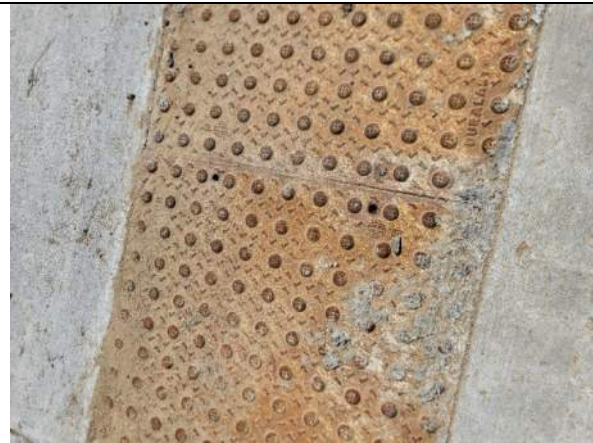
Concrete Clean up/seal all ADA ramps
