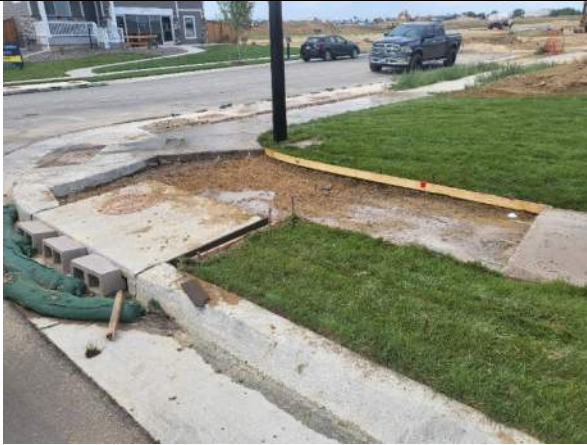
Concrete Item (Hole was full of water)
