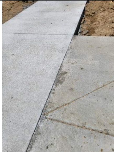
Concrete Clean up
