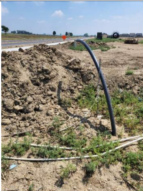
Utilities covered with peds Clean up
