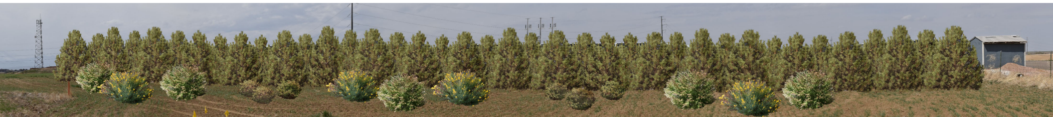
Substation with screening
