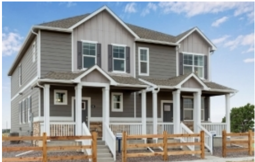
REAR LOADED DUPLEX HOMES
