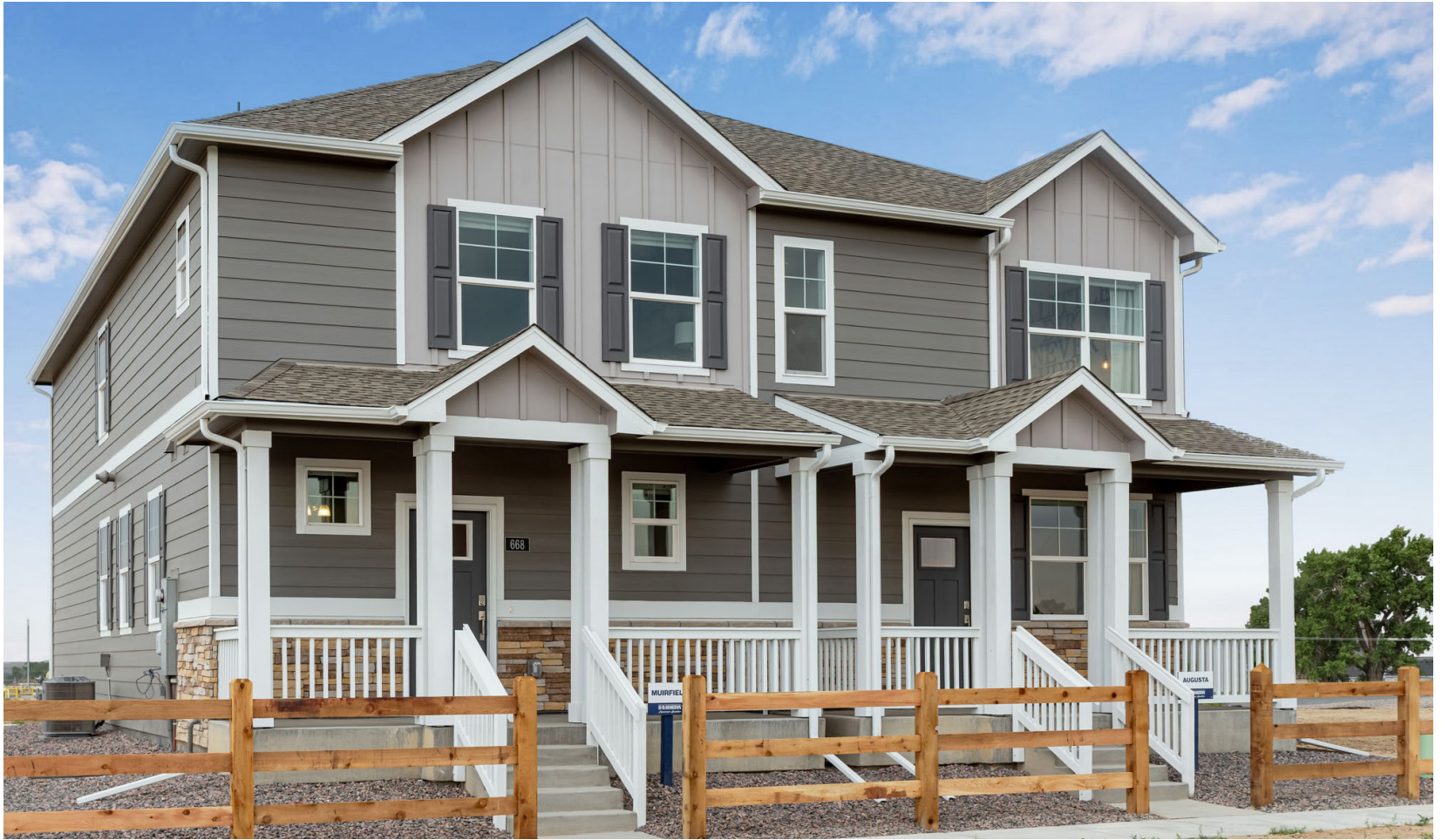
REAR LOADED DUPLEX HOMES
