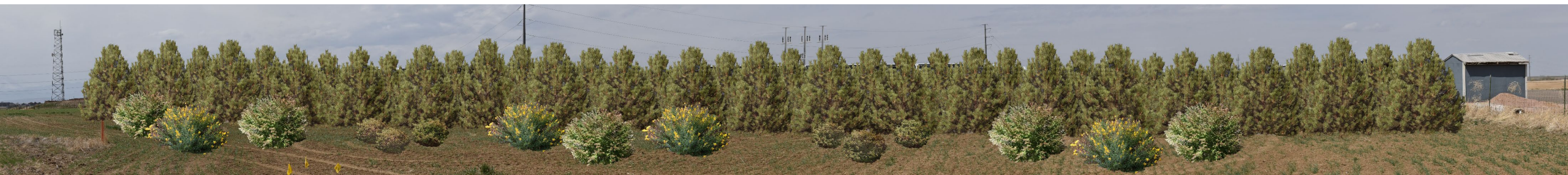
Substation with screening
