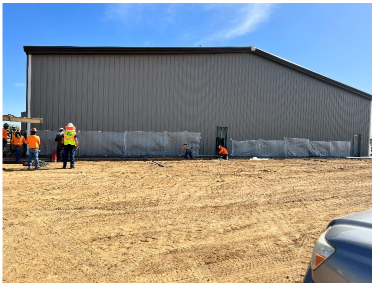
Site concrete paving placement north side of building
