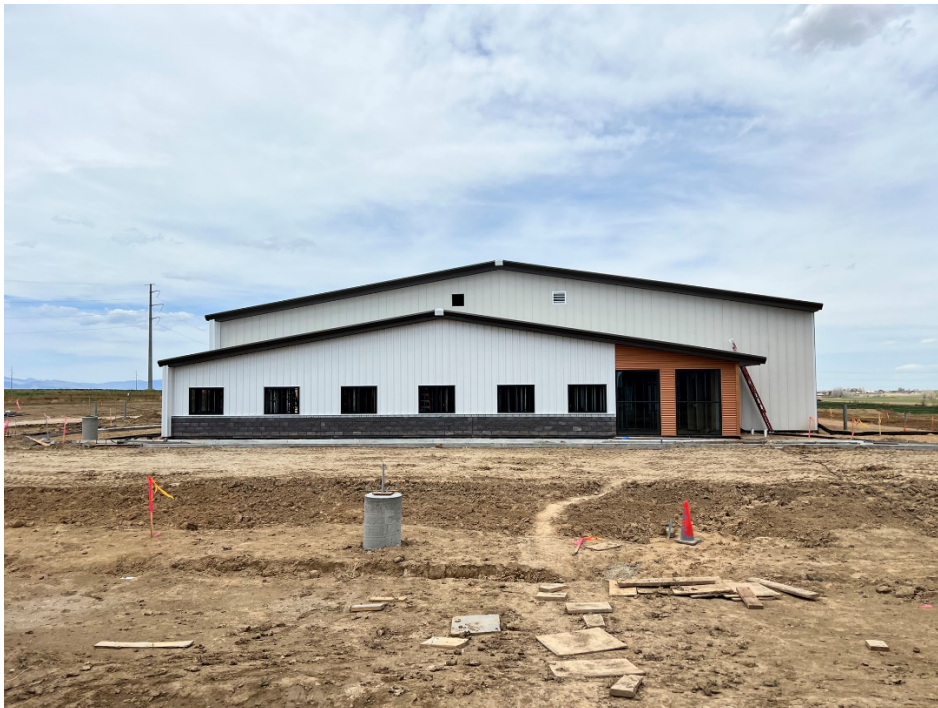
South Side Elevation Construction Progress
