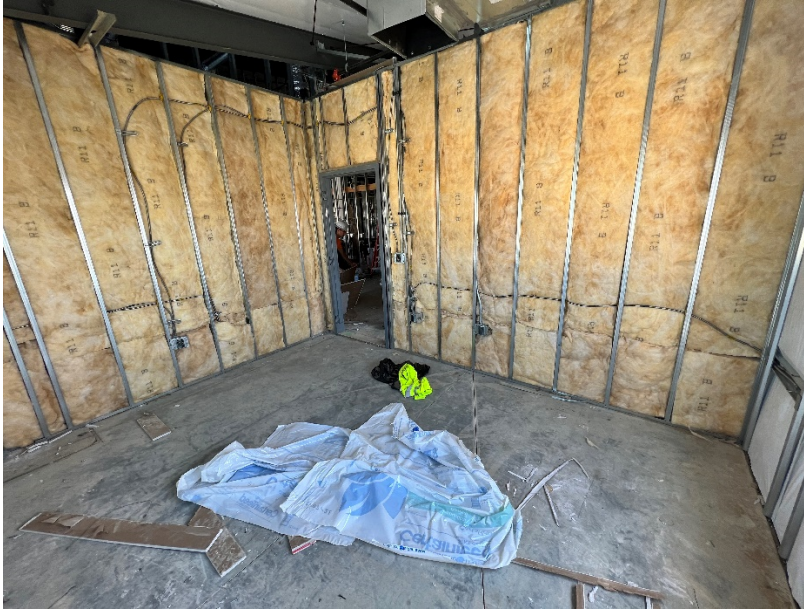
Interior wall and insulation installation
