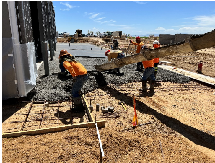
Site concrete paving placement west side of building
