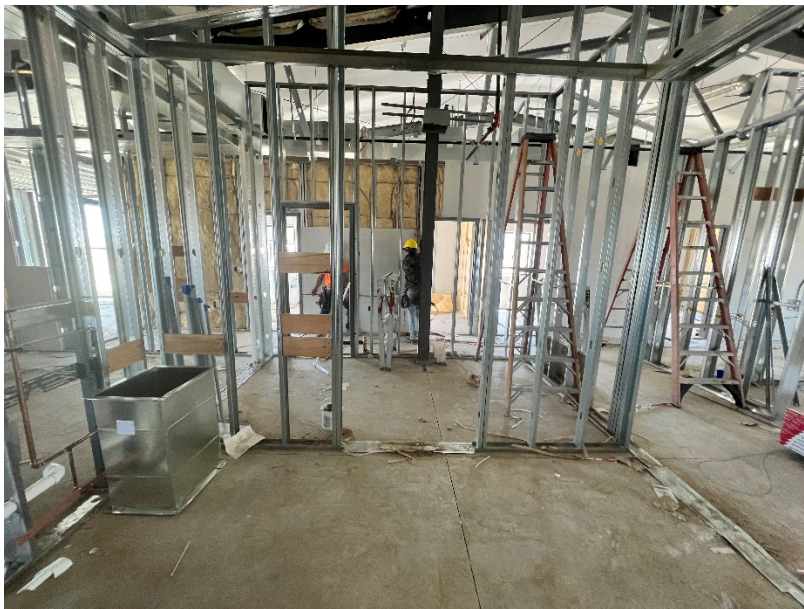
Interior wall construction
