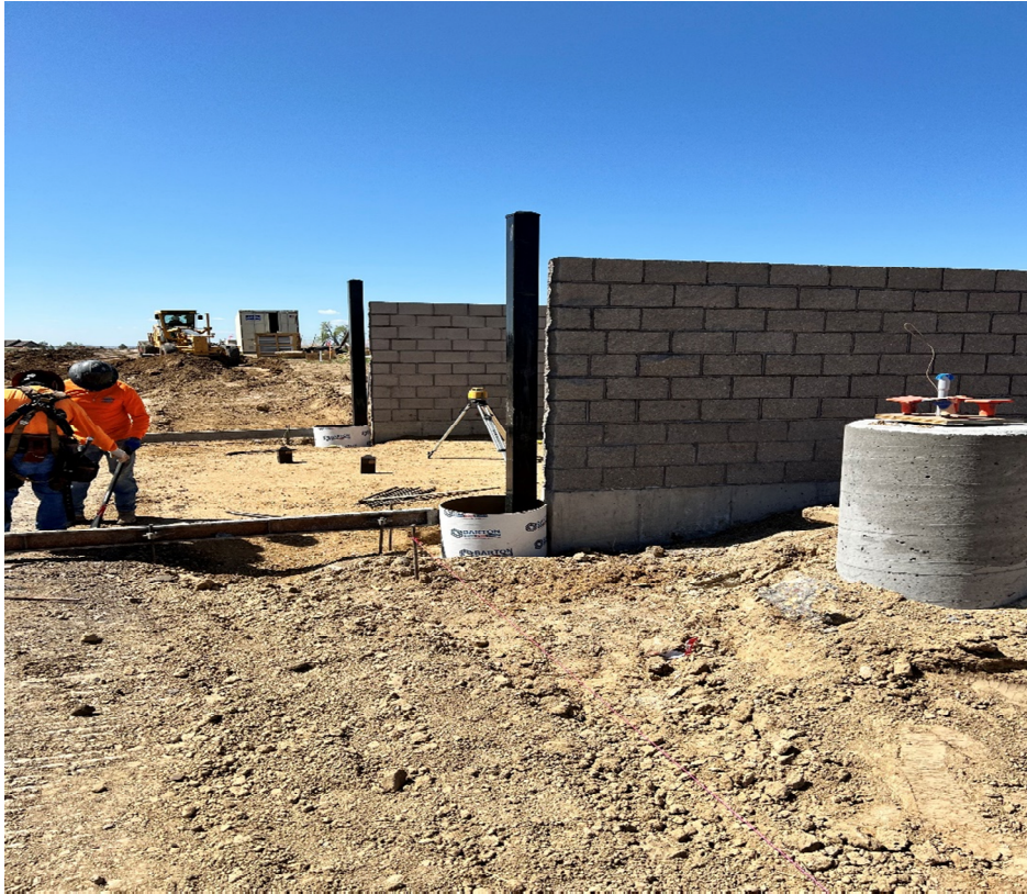
Trash Enclosure Construction Progress
